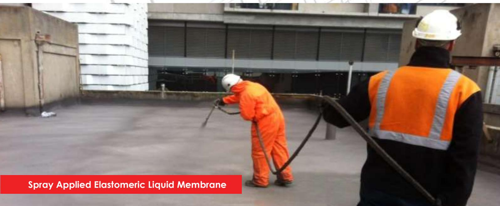
Spray Applied Elastomeric Liquid Membrane
