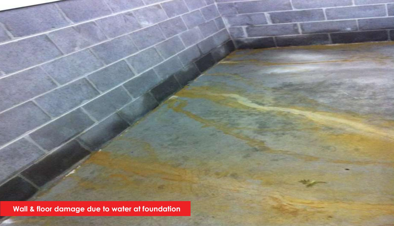
Wall & floor damage due to water at foundation
