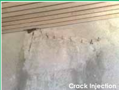
Crack Injection
