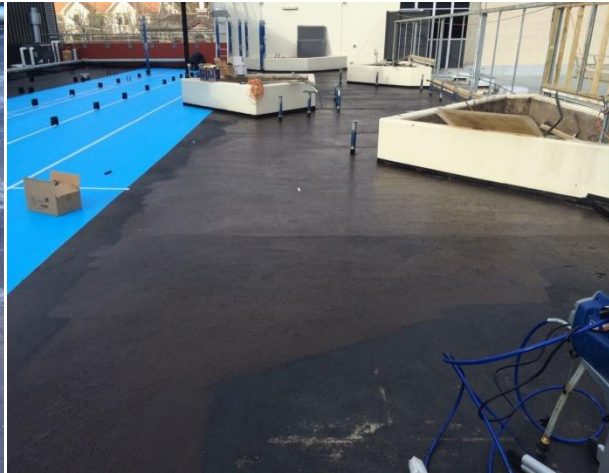
Finished membrane with protection sheet prior turf
