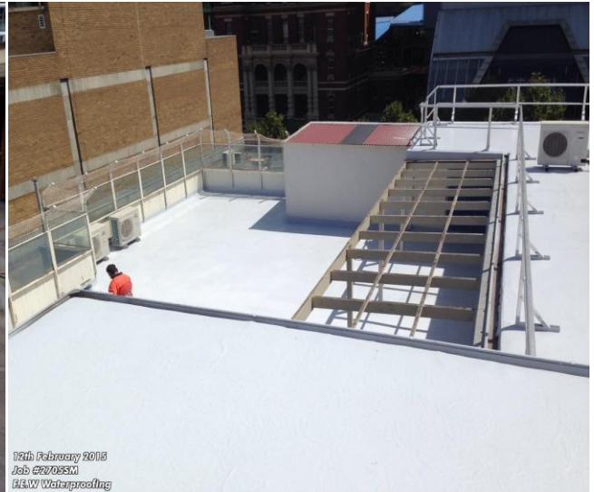
Finished roof surface with Thermo Top Coat
