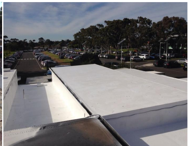
Spray Apply Liquid Waterproofing
