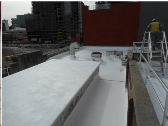
Finished roof surface with Thermo Top Coat
