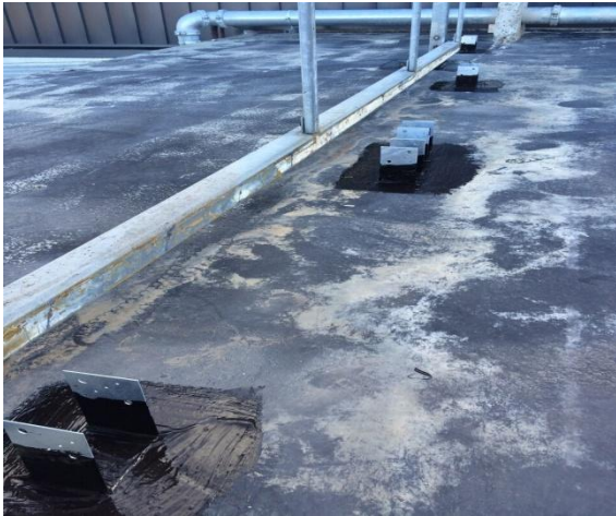
Existing roof surface
