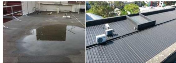
**Rooftop deck with water ponding causing catastrophic structural damage to the building.**
