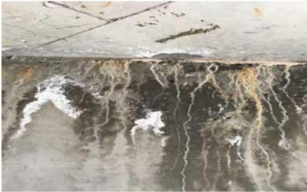
**Extensive concrete damage to underground car park due to water leaks from rooftop above.**
