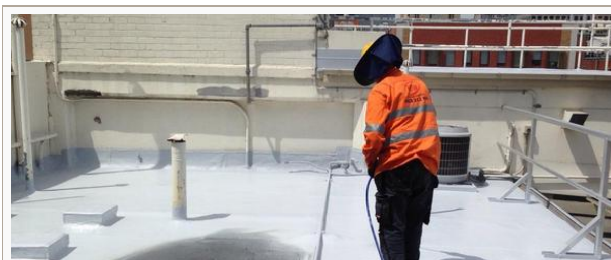
Spray apply reflective white top coat
